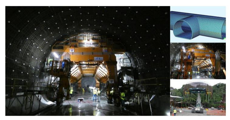
The Changuinola Hydroelectric Plant, located in the Bocas del Toro province in Panama, includes a 4,1 km long pressure headrace tunnel (HRC) and a 450 m long surge Adit tunnel (SA).
